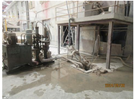
Slurry and Mud Making Workshop.JPG
